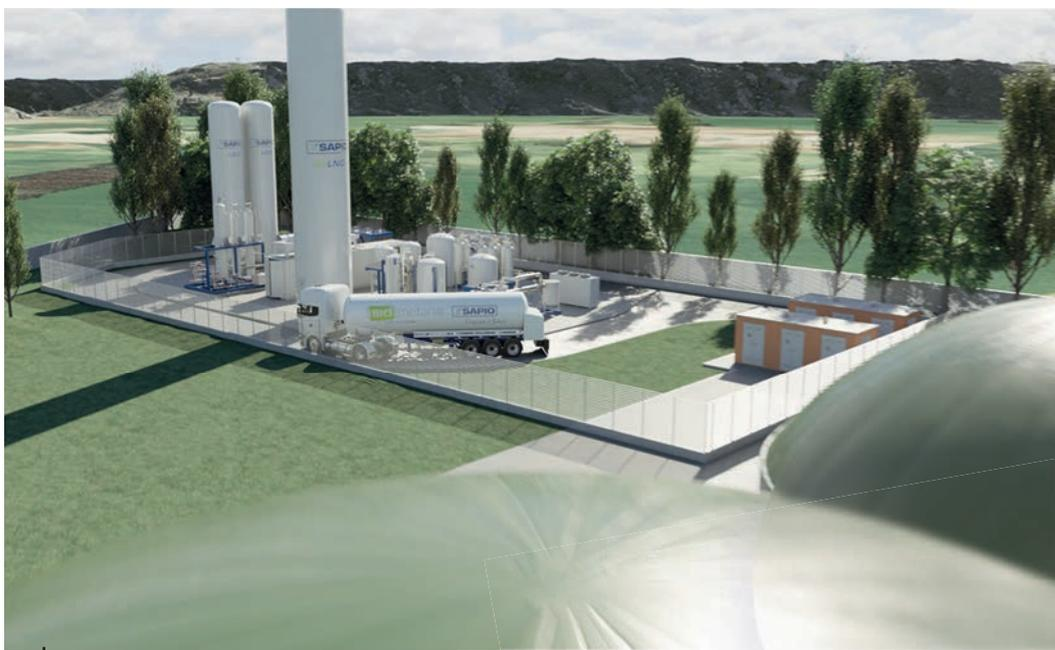
*Sapio supplied a first upgrading plant with PSA (Pressure Swing Adsorption) technology to the Assoro Biometano Agricultural Company in Sicily, one of the very first biomethane production projects in the agricultural sector in Italy.*
